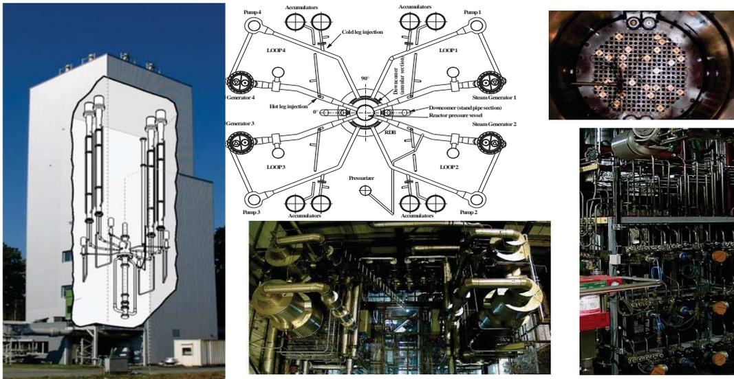
Figure 4: PKL Loop – left: photo of the building with a scheme of the main components – center top: scheme of the arrangement of the main components – center bottom: view into the loop from the bottom right top: photo view in the core mock-up – right bottom: photo of pressure transducer arrangement
